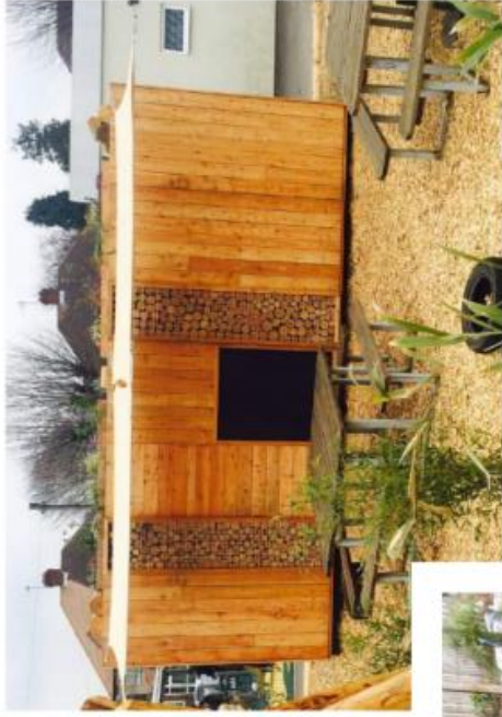
A shipping container provides a large secure storage space. The timber cladding creates an attractive facade with integrated insect habitats. Other features include a green roof and sail shades, which provide a sheltered space for seating and an outdoor cooking area.
